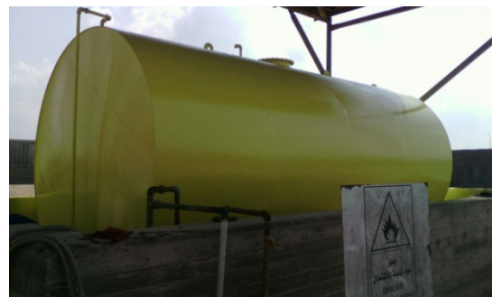
Sandblasting & painting of solar tanks-Danone Farm
